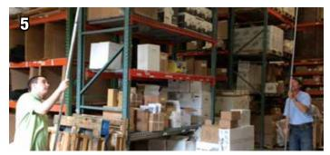
With one person on each end, carefully lift the extension poles and walk the net assembly to the target area. Once in the correct area, lift the extension pole and attach the tip to a rafter or other structure. Or use the hooks provided in the kit if the magnetic adapter is not appropriate. FOR SAFETY: DO NOT LEAVE THE HANGING NET ASSEMBLY UNATTENDED.
