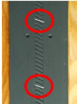
**3.7** In most cases it is best to secure the proofing strip with suitable flat-headed screws e.g. 3/4-1 inch (20-25 mm) long No. 10 (4.8 mm) hex head screws or pan head screws with a No. 2 Philips recess. For mounting on sheet metal doors, the screws should be self-drilling sheet metal screws.
