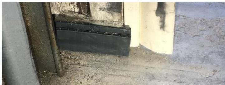
Two layers doubles the effectiveness of the protection against rodents. Two layers are therefore recommended where the rodent pressure is high.
