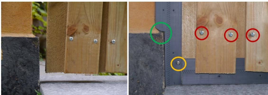
The screws in every second board (the 3 red circles) were loosened and the horizontal proofing strip was tucked in between the boards. Thereafter the screws were retightened.
