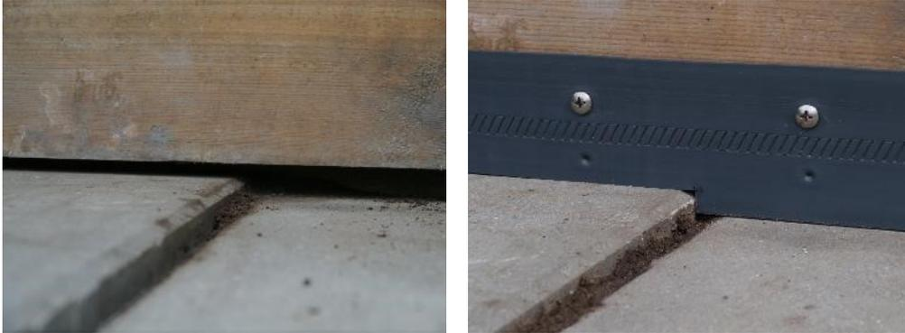
It was easily adapted by means of straight tin snips and a Stanley knife.
